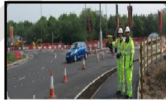
ROAD SAFETY AUDIT
