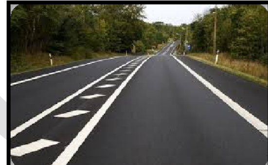
THERMOPLASTIC ROAD MARKING
